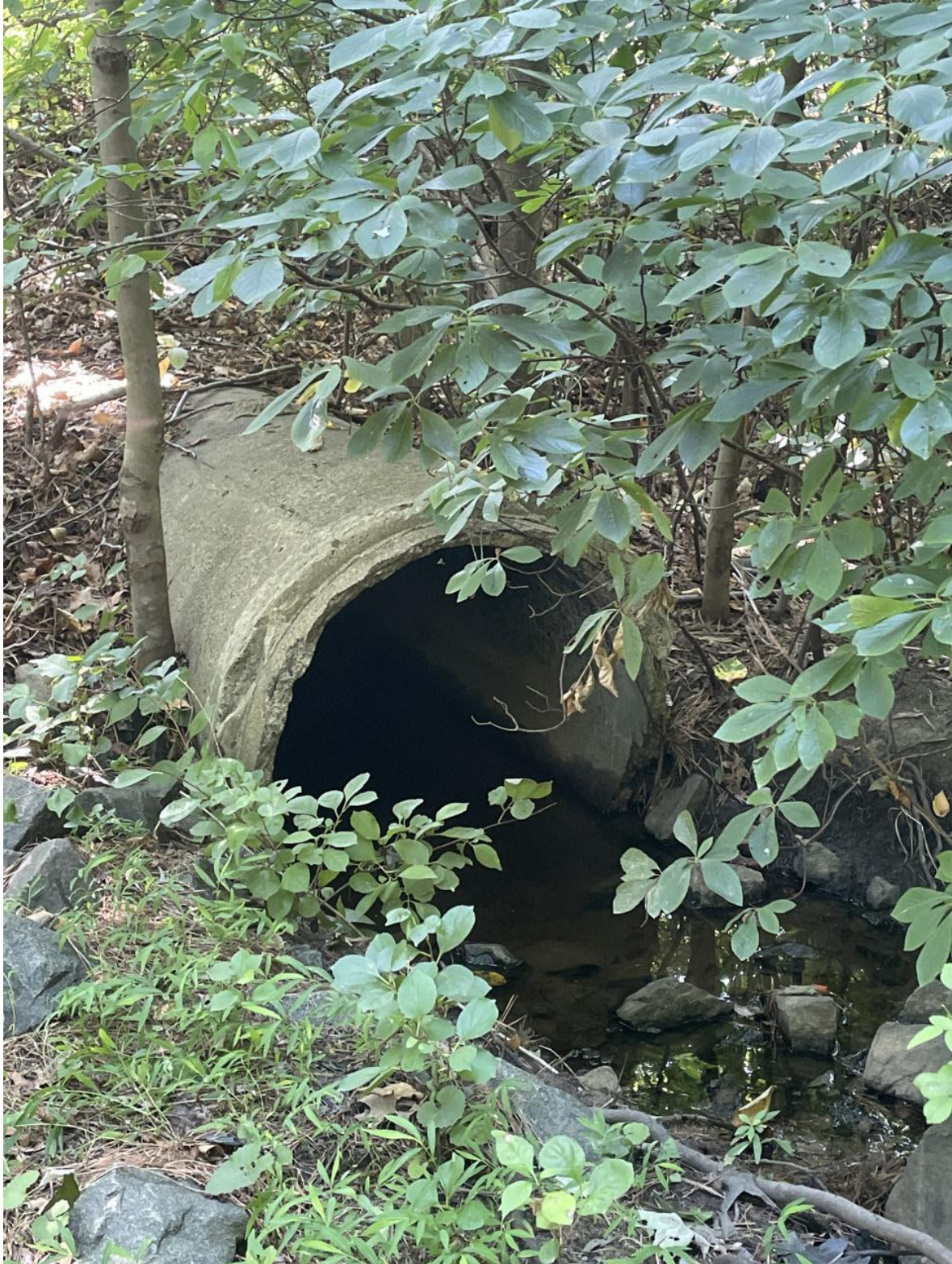
Outfall ID: AC02 (8/4/2022)
