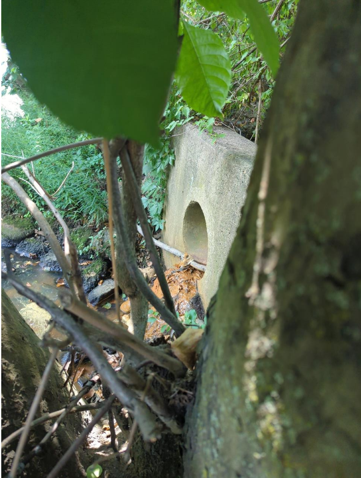
Outfall ID: AC14 (7/22/2022)
