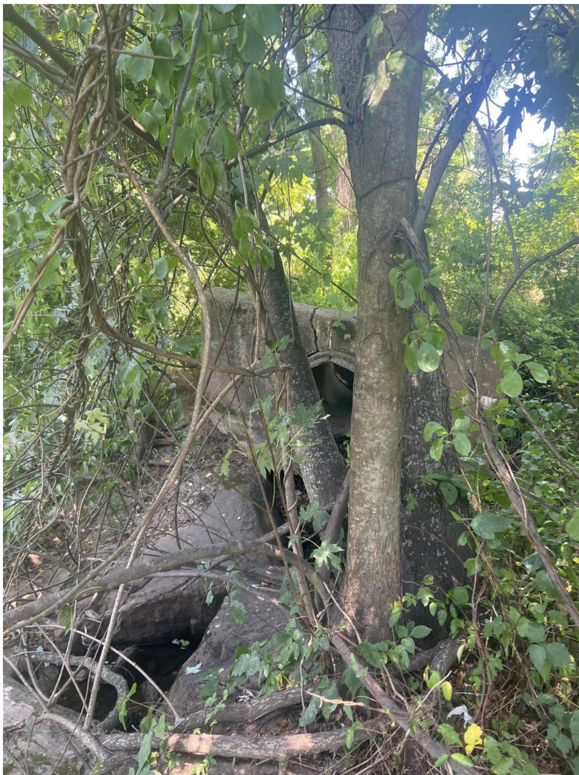
Outfall ID: AC09 (7/22/2022)
