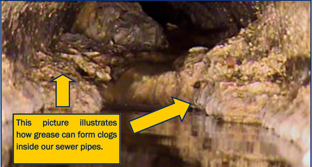
This picture illustrates how grease can form clogs inside our sewer pipes.
